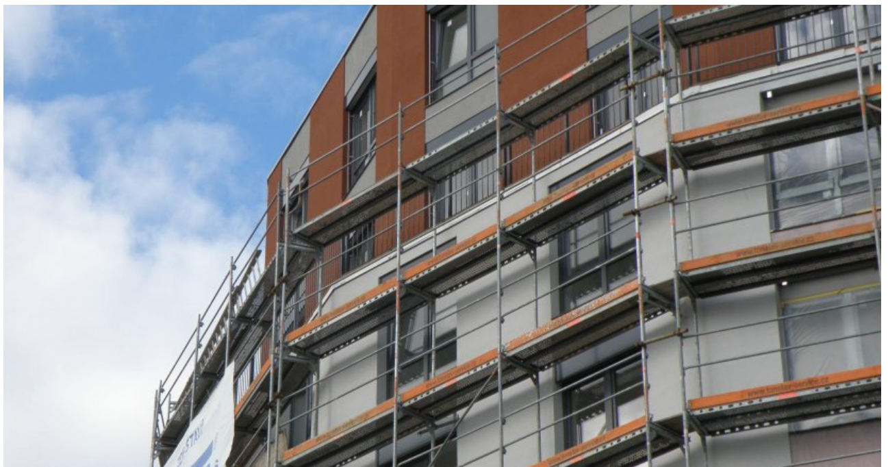
External isolation in a building © Pixabay
